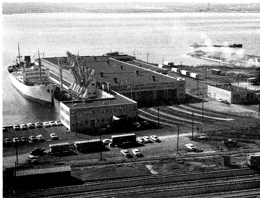
BALTIMORE . . . The B&O Railroad's modern fruit pier at Locust Point is the site of the annual discharge of more than 4 million stems of bananas annually. Approximately two United Fruit Line ships visit the pier weekly. Completely air conditioned, the new $4.3 million pier has modern conveyor systems which permit the simultaneous loading of 63 railroad cars located on 7 undercover tracks. The motor truck area provides covered space for 42 trucks and an additional 12 out-of-doors. Preheating yards adjacent to the terminal are capable of controlling the temperature level in as many as 180 rail cars prior to loading.
