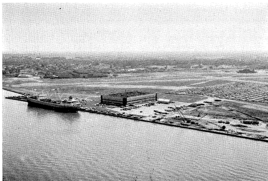
Dundalk Terminal, the newest marine terminal in the Port of Baltimore, opened to receive the first ship ever to dock at the former airport on January 4, 1960. The 353 acre site was bought from the city in November, 1958. Repairs have been made to the former seaplane hanger and to the bulkhead, and a 20 acre plot of land has been paved, lighted, and fenced for an importer of foreign cars, the first tenant. The Maryland Port Authority took possession of 126 acres on January 1, 1960, and will assume ownership of the remaining land on January 1, 1961.
