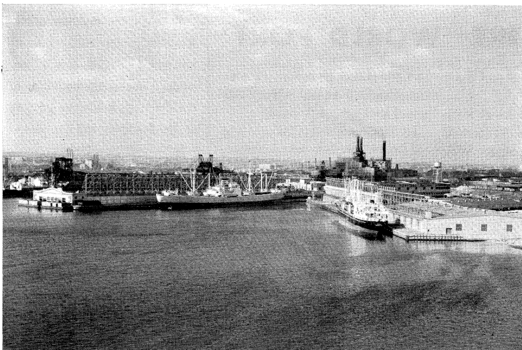
BALTIMORE . . . The Port Covington terminal of the Western Maryland Railway includes 5 covered piers, 2 open piers, a coal pier, new modern ore dock equipped with two highspeed unloading machines and automatic weighing devices and grain elevator. The facility can unload 27 vessels simultaneously.
