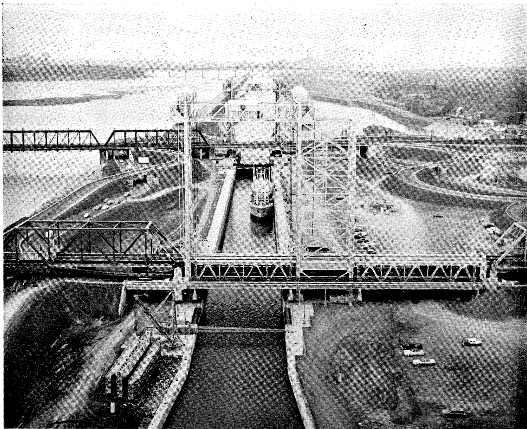
The St. Lambert Lock , the most easterly of the seven new Seaway locks. Alike the other six locks, this one is 768 feet long, 80 feet wide with 30 feet of water above the sills. Ships enter the Seaway a short distance downstream of the Jacques Cartier Bridge seen in background. In middle-ground are the two vertical lift spans of the Victoria Bridge which, through alternate use, provide uninterrupted traffic on the bridge while a ship is in the lock. Also in background is a portion of the 20-mile long channel which extends from the entrance in the Montreal harbour to Lake St. Louis, upstream. This channel has a minimum width of 200 feet. Lift of the lock is 15 feet.
