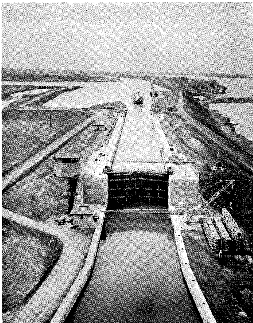
Pictured here is the Cote Ste. Catherine Lock, one of two locks in the Montreal area of the Seaway. It is built overland to by-pass the Lachine Rapids (out of sight on the right) long considered the natural barrier to navigation on the St. Lawrence River. Lift of this lock is some 30 feet. Although some 20,000,000 gallons of water are required to fill the lock, this is done in less than 10 minutes.
