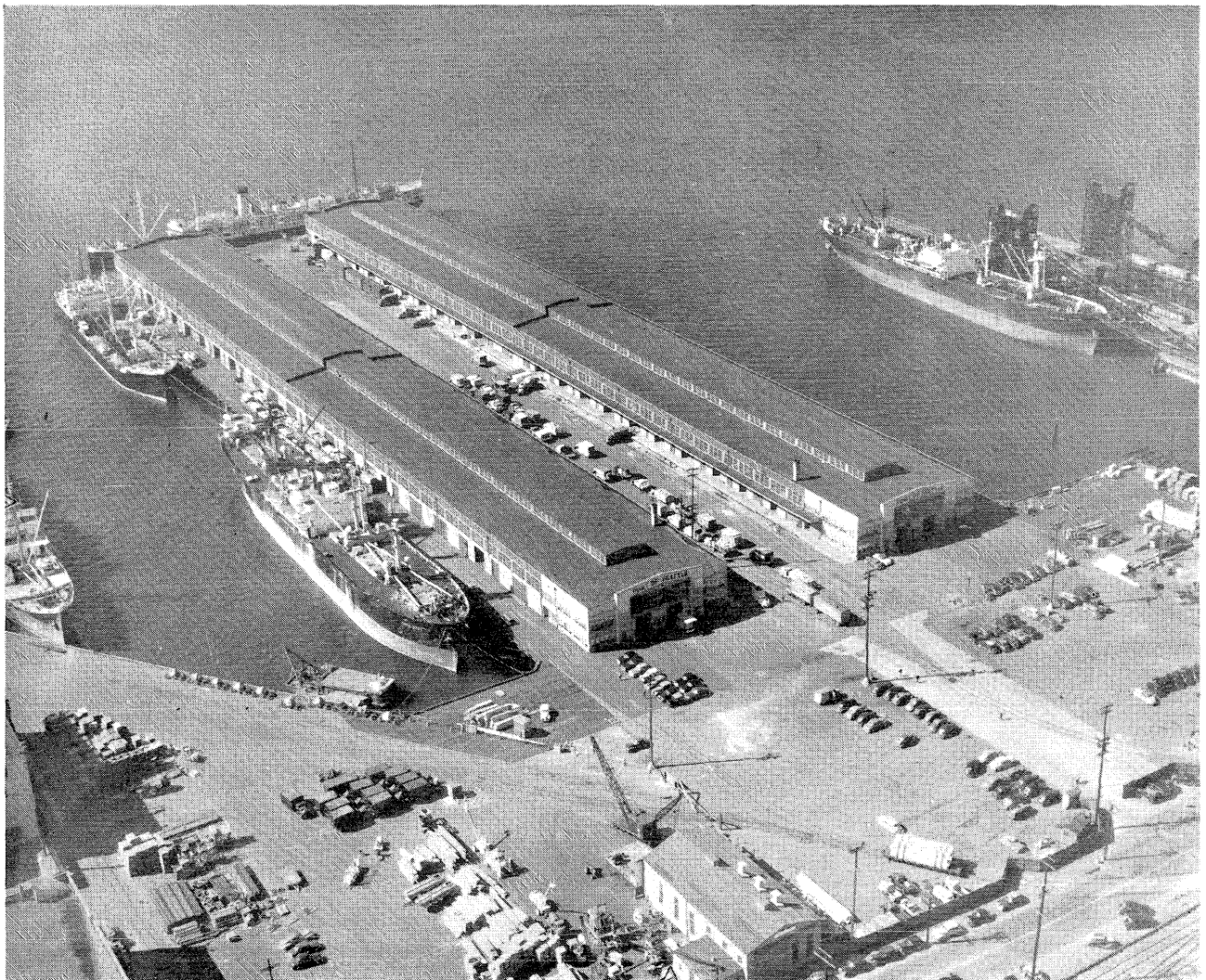
Pier 42, owned by the Port of Seattle and leased to the Alaska Steamship Company. Pier 42 is 1102 feet by 396 feet, and has 215,820 square feet of covered storage area, and open storage area for 40,000 tons.
