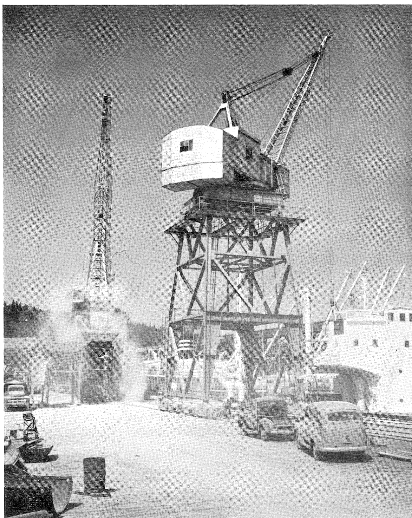
Two gantry cranes at Terminal No. 4 unload zinc concentrates. Each crane is capable of handling 125 tons per hour of ores or concentrates. Cargo can be loaded either into open stockpiles or directly into trucks or rail cars with these cranes. Terminal No. 4 is one of the most modern bulk cargo terminals on the Pacific Coast.
