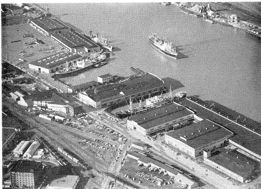
Aerial view of Terminal No. 1 of the Commission of Public Docks. This 46-acre general cargo terminal provides the most modern handling and storage facilities available to maritime commerce. Direct dockside rail loading is provided at all piers and ample open or closed storage area is always available. This terminal provides a 100-ton shear leg crane for heavy lifts.
