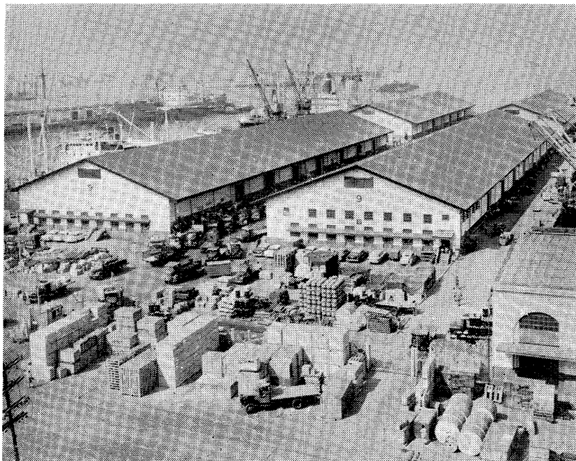
Pier 9 is well adapted to the needs of modern shipping. It has 2 gantry cranes on each apron with tracks running along the whole lengths of the cargo sheds. Shed B, on the right, is ideal for the discharging of vessels with a big volume of cargo because of its proximity to Pier 7 where cargo overflow can easily be shifted for storage.
