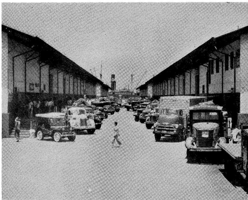
This depressed roadway at the center of Pier 9 facilitates the loading of trucks with the use of a minimum number of delivery equipment. This feature enables the serving of three trucks simultaneously at each delivery door.
