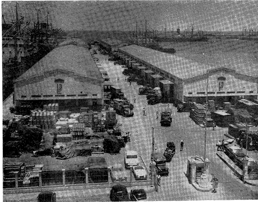
Pier 13 replaced the destroyed two-story Pier 7 of prewar renown. It is longer than Piers 9 and 7 and can take in vessels of deeper drafts. Its eleven- and ten-door cargo sheds make possible the simultaneous delivery and fast turnover of cargoes.
