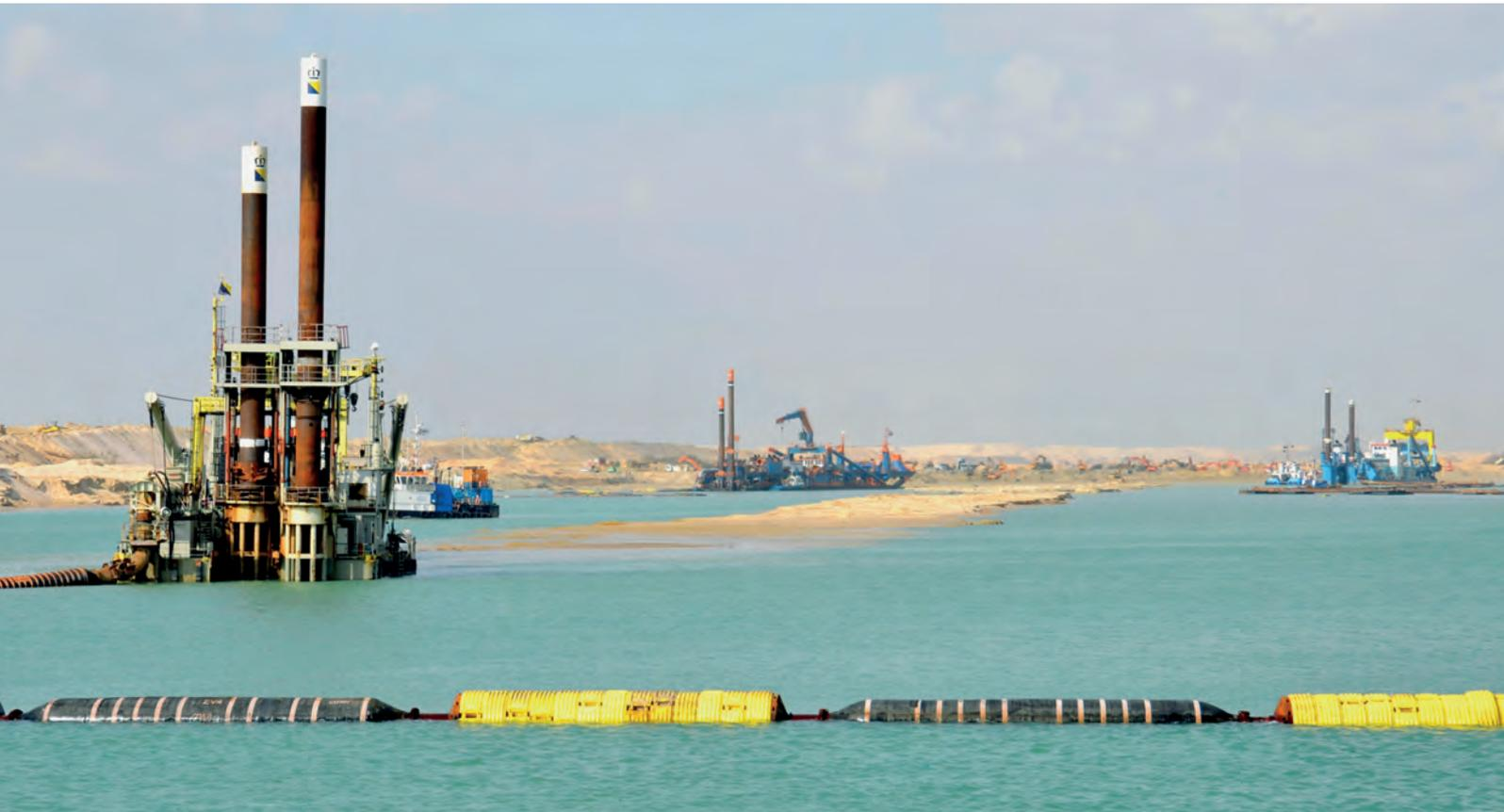
Picture: Ismailia, Egypt – dredging for a new waterway to expand part of the Suez Canal in 2015. The works converted part of the one-way canal into a two-way stretch. Photo: Alamy/BJ Warnick
