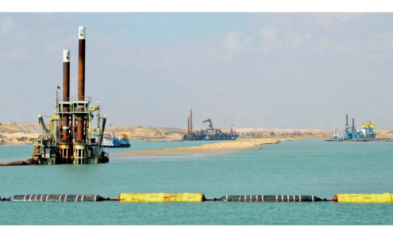
Picture: Ismailia, Egypt – dredging for a new waterway to expand part of the Suez Canal in 2015. The works converted part of the oneway canal into a two-way stretch. Photo: Alamy/BJ Warnick
