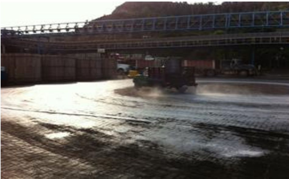
Moisturization and application of biodegradable product on waterways for control of resuspension of the material by the traffic of vehicles.
