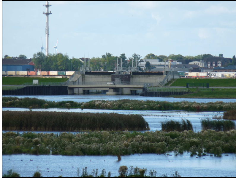
Storm flood barrage and tidal polder at high tide (Photo: Uwe von Bargaen)
