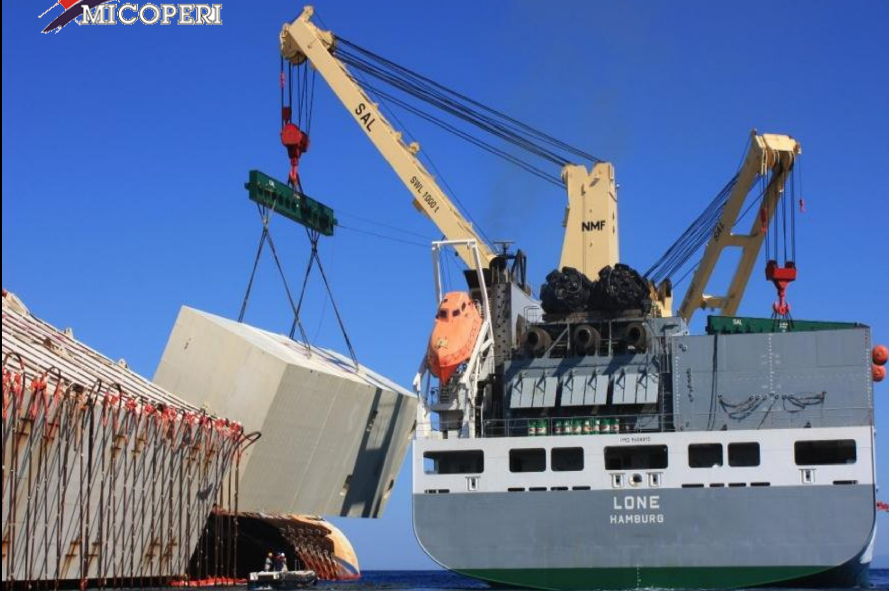
HEAVY LIFT VESSEL FOR SPONSON INSTALLATION
