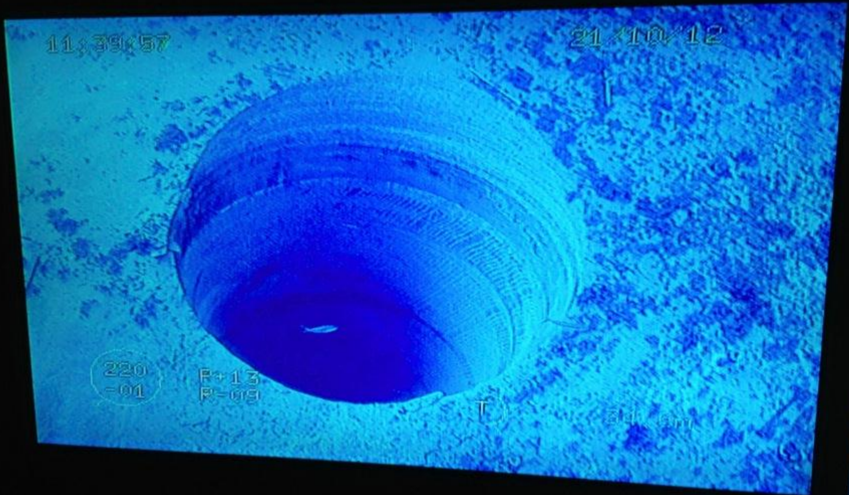
2 M DIAMETER DRILLING ON GRANITE - PLATFORM LEGS
