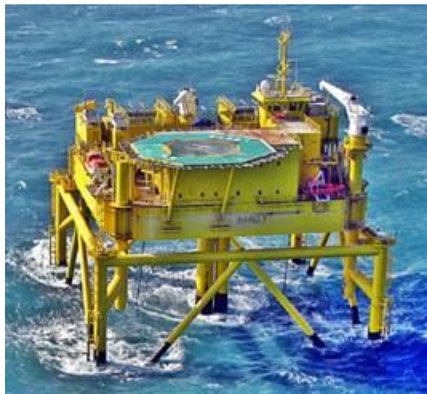
Figure 12 Accommodation Facilities on the Transformer Substation of the OWF “BARD Offshore 1”
