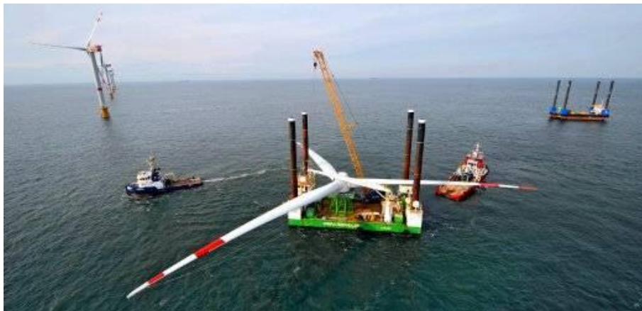
Figure 5 Jack-up Platform transporting pre-assembled Rotor Star
