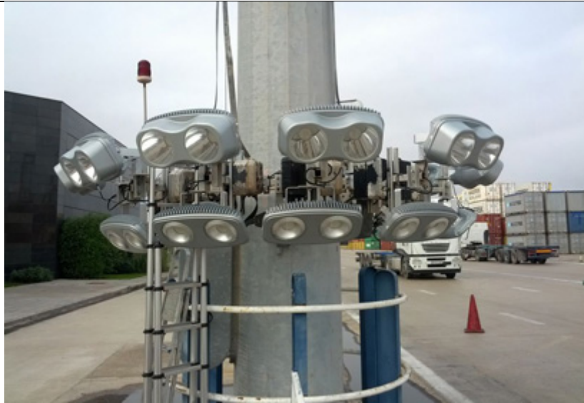
LED Luminaires installed at Noatum Container Terminal Valencia
